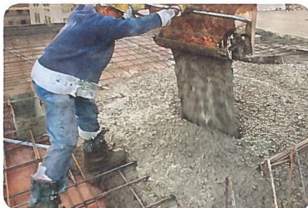
Figure 4 Steel reinforcing bars (rebar) serve to strengthen concrete by allowing it to resist both tension and compression.
