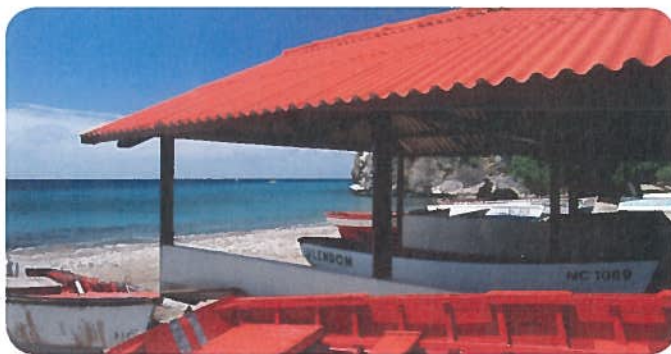
Figure 3 The corrugation in a steel roof provides added strength.
