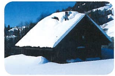
Figure 4 The steep shape of this chalet roof allows heavy snowfalls to slide off.
