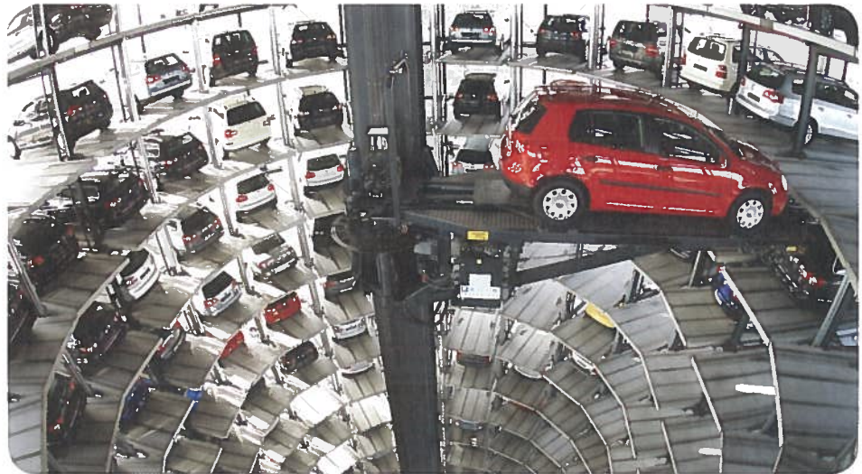
Figure 1 The VW Autostadt structure in Wolfsburg, Germany, stores cars until the automated system retrieves them.
