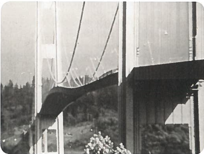
Figure 1 Blowing wind resulted in the torsional twisting of the Tacoma Narrows Bridge, photographed shortly before its collapse.
