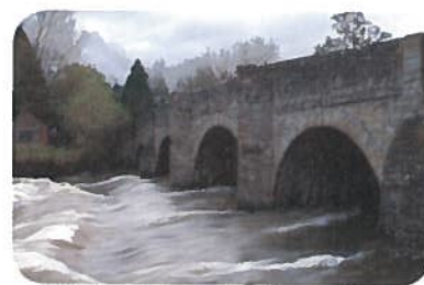
Figure 9 Rushing water striking a bridge is an example of a dynamic load.
