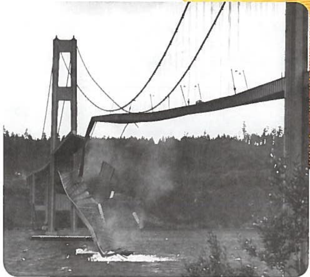
Figure 2 The collapse of the Tacoma Narrows Bridge
