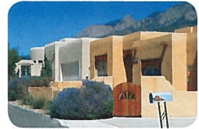
Figure 5 The flat roofs on these adobe homes work well in areas with very little rainfall.
