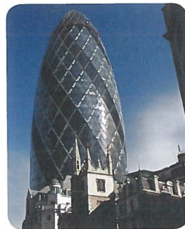
Figure 3 The St. Mary Axe building in London, England, shows its frame structure.
