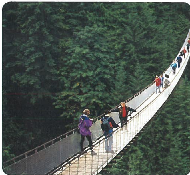
Figure 4 The main cables in a suspension bridge, like the Capilano Bridge in British Columbia, have tension forces acting on them.
