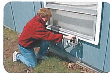
Figure 5 Weather stripping reduces drafts and energy loss.
