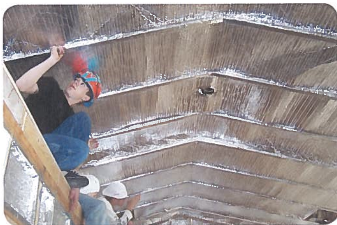
Figure 7 Radiant barriers are generally installed in the attic of a house to minimize energy transfer into the home.
