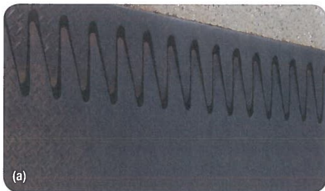
Figure 2 (a) The expansion joints narrow when bridge segments expand in hot weather. (b) Expansion joints in a bridge separate when the side-by-side segments of a bridge contract in cold weather.
