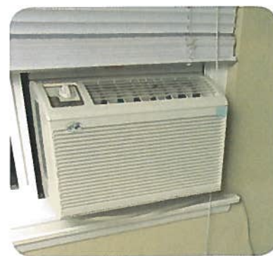
Figure 3 Air conditioners are often fitted into building windows, where they draw in outside air, cool it, and blow it back into the building.
