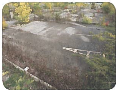
Figure 1 This parking lot has become overgrown with vegetation.
