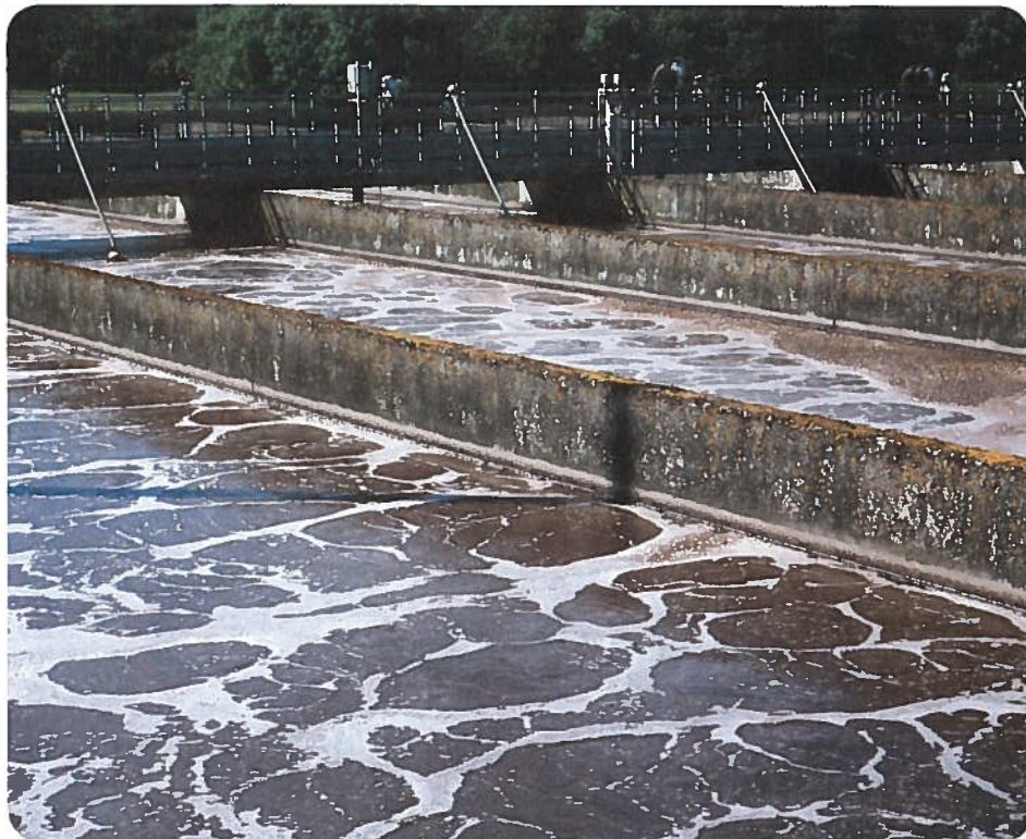
Figure 2 During secondary treatment, bacteria remove any wastes left in the liquid mixture.
